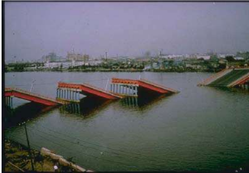
Figure 1 - The breakdown of the Schwaukee Bridge in the Niigata earthquake (Bhattacharya, 2003)
